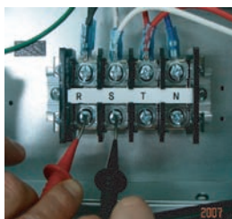
* Measuring input voltage
