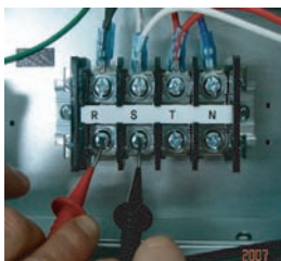
* Measuring input voltage
